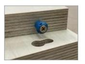
**Insert the Peanut** Use a mallet or hammer to insert the Peanut flush
